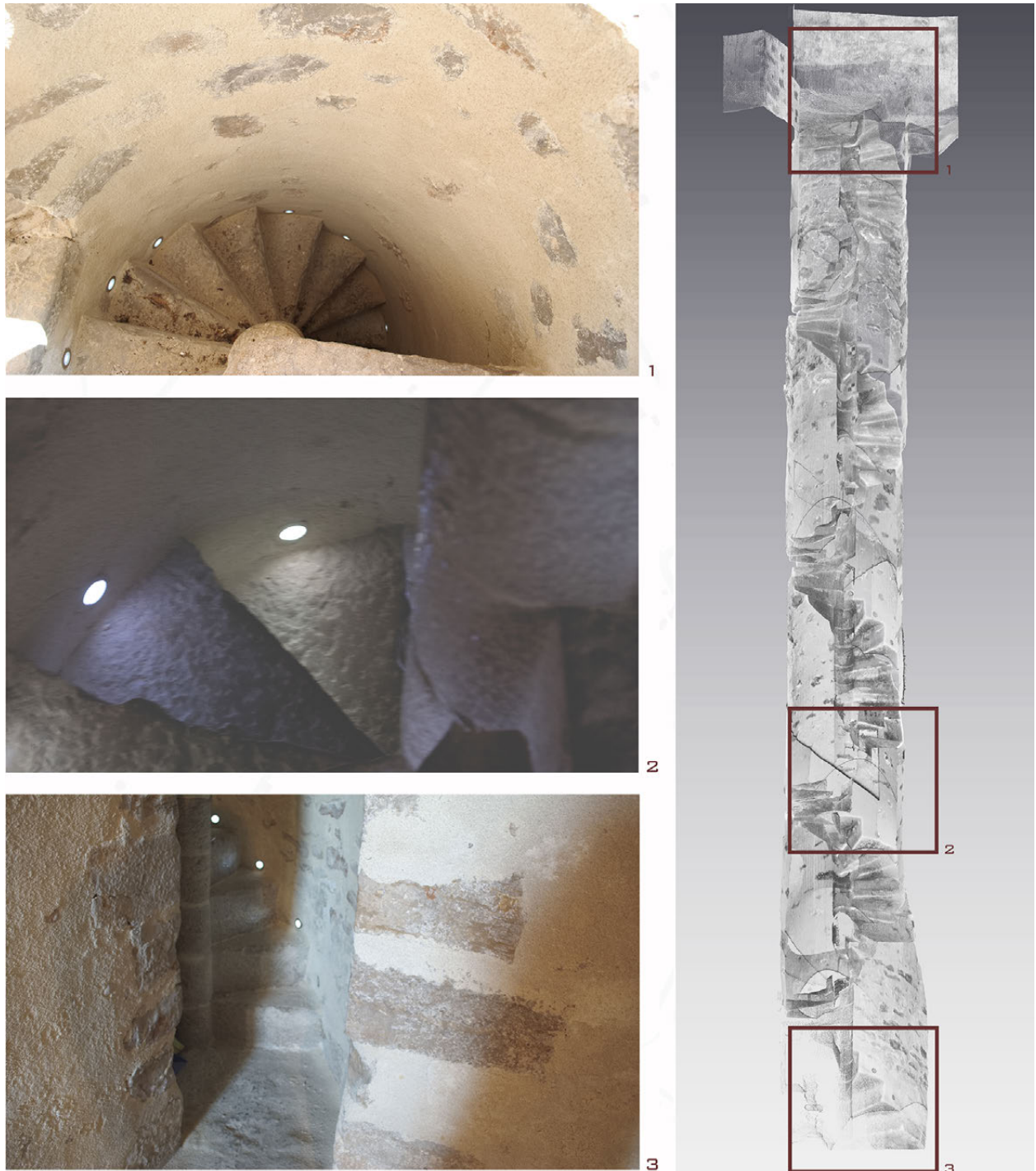
Figure 7. Spiral staircase with a central pillar.
