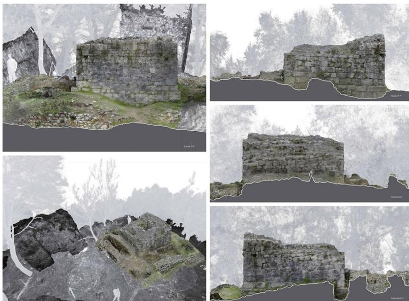
Figure 11. Results from the photogrammetry: the northern tower, sections.
