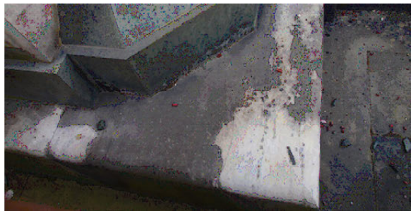
Figure 15. The white marble erosion.
