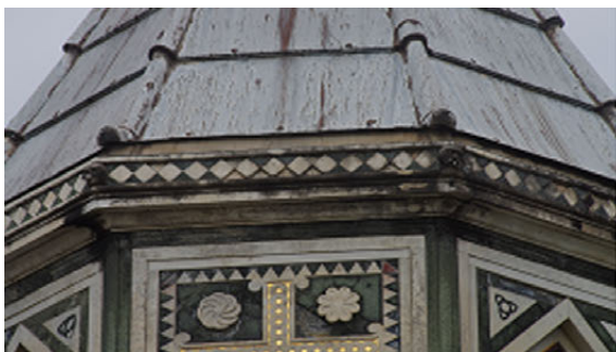
Figure 10. Lead on roof.
