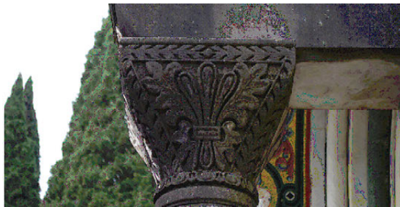
Figure 14. Disintegration in Verde Prato.
