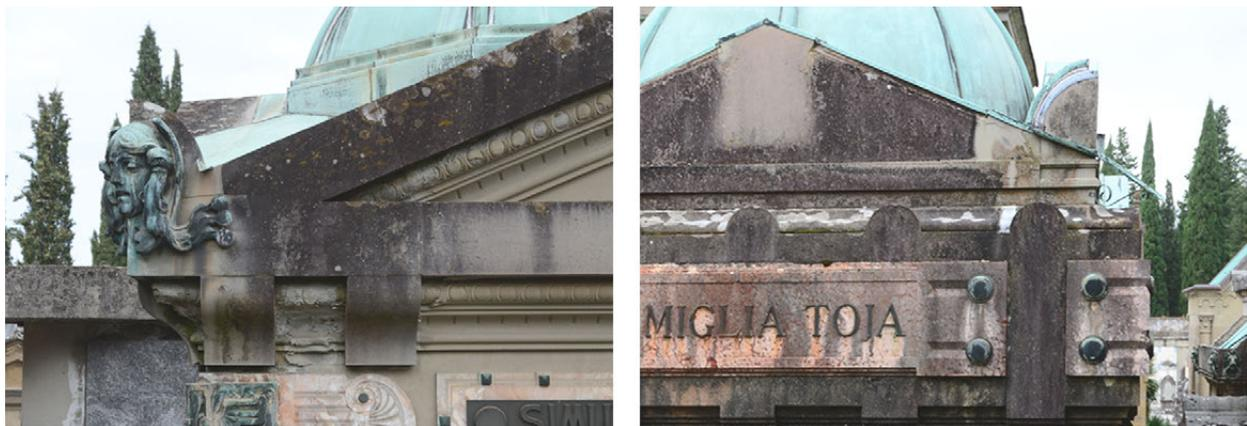
Figure 12. The roof covering and its related degradation: Bartolani on the left and Toja on the right.
