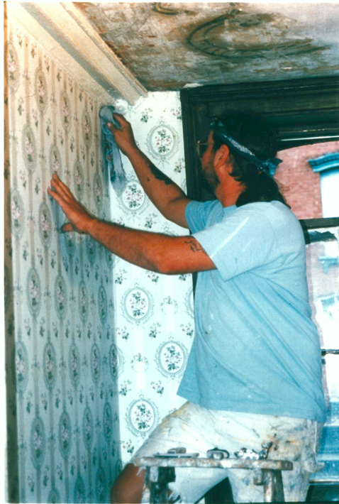
Figure 7. Restoration carpenter Kevin Groves installs reproduction wallpaper in the Gumpertz Family Apartment, 1994. Courtesy of the Lower East Side Tenement Museum.
