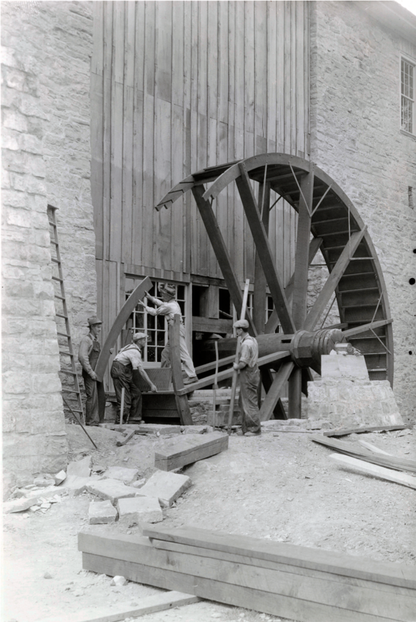
When Indiana Department of Conservation workers restored the mill at Spring Mill State Park in 1930, they built a new vertical wooden waterwheel. The mill's original wooden wheel had been abandoned decades earlier in favor of a metal water turbine.
