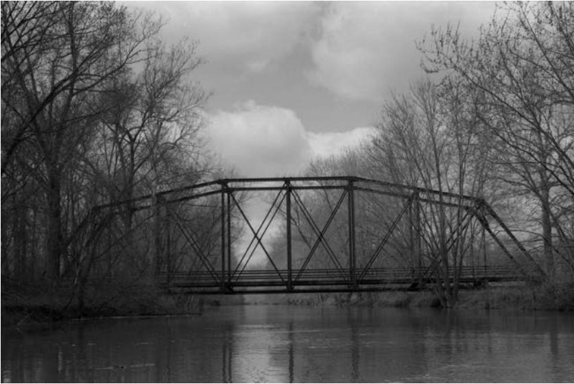
The 1924 Camelback bridge. After completing Houchins Ditch, engineers built this bridge to allow passage across the sixty-foot-wide channel.
