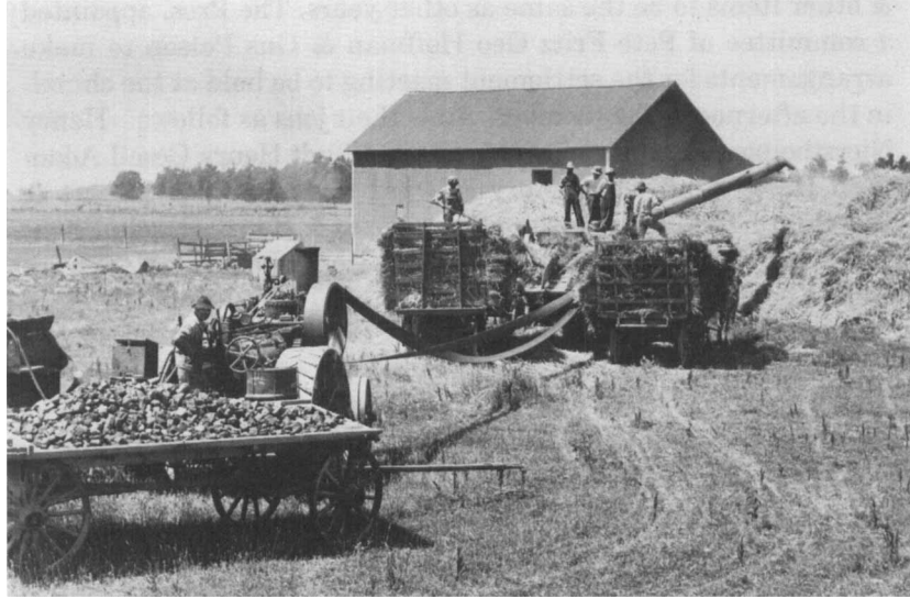
A COAL BURNING ENGINE FIRES THE SEPARATOR IN THIS EARLY TWENTIETH CENTURY INDIANA THRESHING PICTURE. IN MOST THRESHING RINGS, INCLUDING THE WHITE PLAINS RING, EACH FARMER HAD TO SUPPLY THE COAL OR WOOD TO RUN THE ENGINE AT THE "HOME" FARM. THE BUNDLE WAGONERS ARE UNLOADING INTO A SELF-FEEDER WITH A DIVIDING BOARD DOWN THE CENTER. NORMALLY, HOWEVER, ONLY ONE MAN STOOD ATOP THE SEPARATOR RATHER THAN THE THREE HERE DEPICTED.
