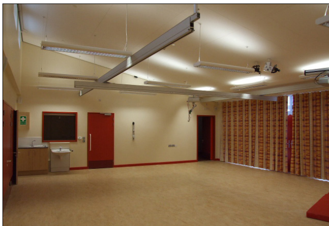
FIGURE 2. Classroom view showing the hoist support beams overhead and the lifting mechanism on the right hand side rear wall.
