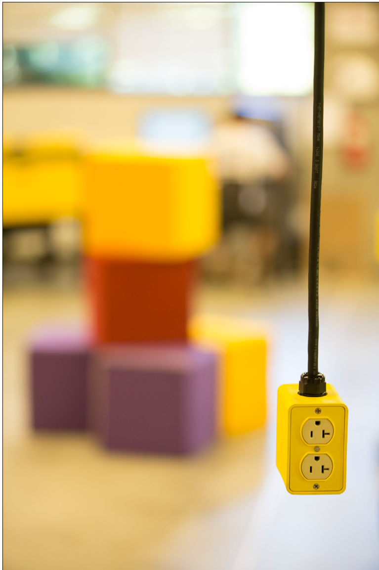
FIGURE 2. These suspended electrical outlets that keep wires off the floor prevent tripping hazards, improve wheelchair accessibility, and allow for flexibility in the space. At the wrong height (and unfortunately as experienced by one of our participants), they can pose problems for people with vision impairments. As an example of a simple change, the CoMotion Makerspace was easily able to reconfigure the location and height of these outlets to maximize access and safety. Credit: Dennis Wise/ University of Washington
