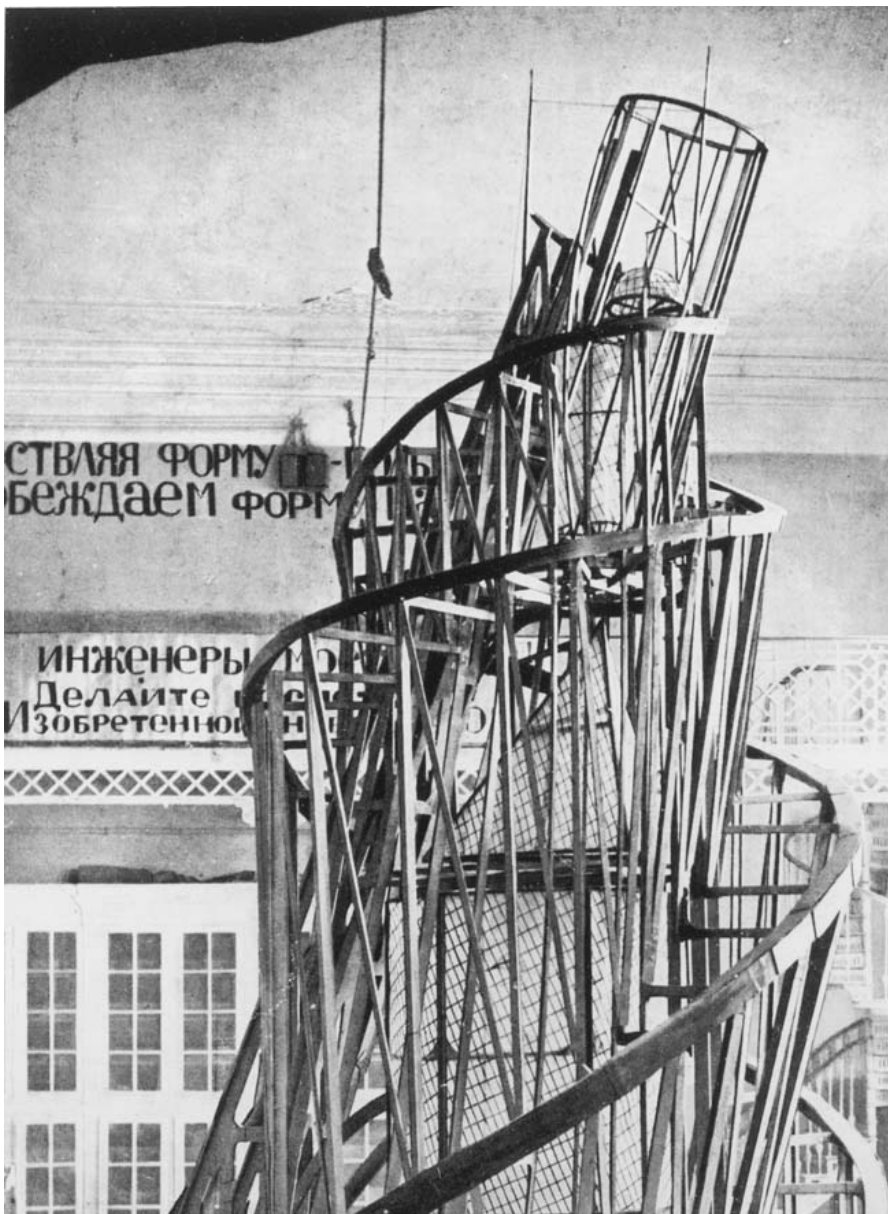
Illustration 3: Vladimir Tatlin's Monument to the Third International (1919-22), a 22-foot-high (6.7 m) iron frame on which rested a revolving cylinder, cube, and cone, all made of glass, which was originally designed for a massive scale, and one of the main monuments of Russian Constructivism. The members of this movement saw themselves as part of the young Soviet revolution, and their projects were intended to contribute to a "construction" of the new Soviet society. In the Constructivists' view, art would directly reflect the modern industrial world. By 1921, Russian artists who followed Tatlin's ideas were calling themselves Constructivists and in 1923 a manifesto was published in their magazine Lef : "The material formation of the object is to be substituted for its aesthetic combination. The object is to be treated as a whole and will be of no discernible 'style' but simply a product of an industrial order like a car, an aeroplane and such like. Constructivism is a purely technical mastery and organisation of materials." The Constructivist artists and architects were committed to complete abstraction with a devotion to modernity. Objective forms carrying universal meaning were considered far more suitable than subjective or individualistic forms.
