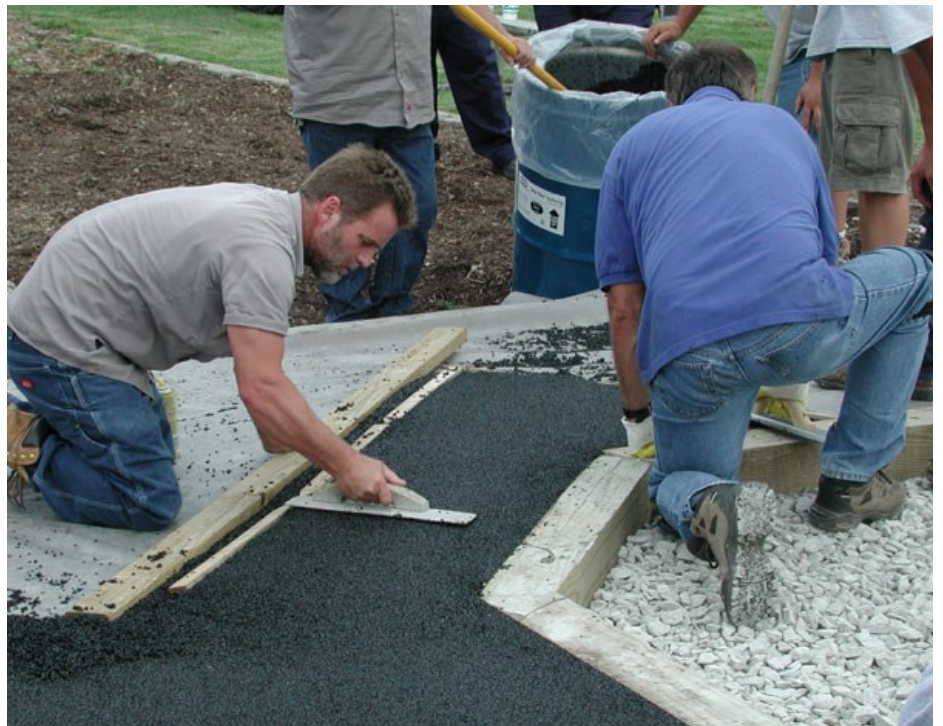
Crews install a playground surface at Thatcher Park in Indianapolis.
