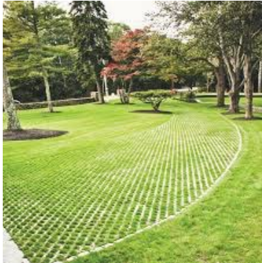
Figure 4. Selected permeable pavers will increase evapotranspiration while remediating water filtration and absorption. (Nicolock Turfstone Pavers, 2020)
