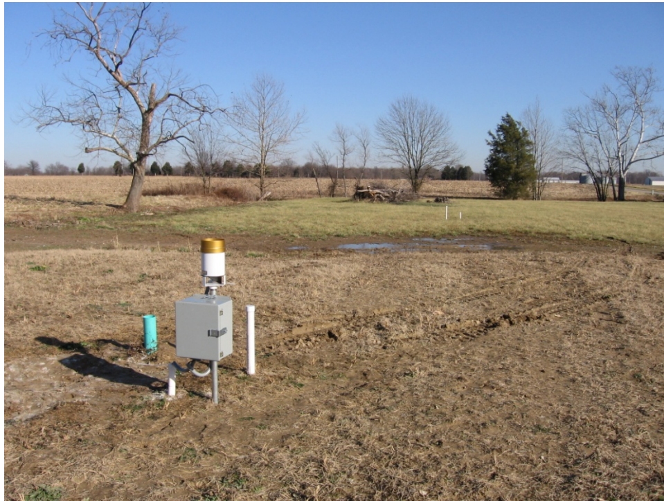
Figure 5. Photograph showing the above-ground instruments installed at the Tire Chip study site.
