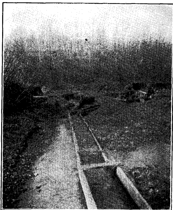
SLUICE-BOXES USED IN SEPARATING GOLD FROM GRAVEL, ALONG HIGHLAND CREEK, MORGAN COUNTY, MARCH, 1903.
