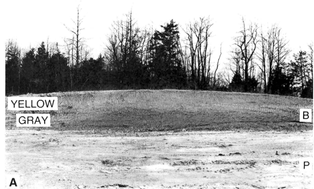
3A. Cross section of the Bethel Formation "B" and upper surface of the Paoli Formation limestone "P" in the area stripped during January 1991. The stripped surface is coincident with the indianaite layer. Cut bank is approximately 6 m high.
