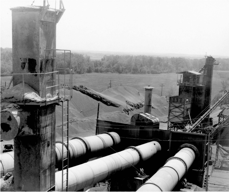
Figure 7. Expanded-shale lightweight aggregate plant of Hydraulic Press Brick, Haydite Div., at Brooklyn, Ind., with three rotary kilns in the foreground and piled lightweight aggregate in the background.
