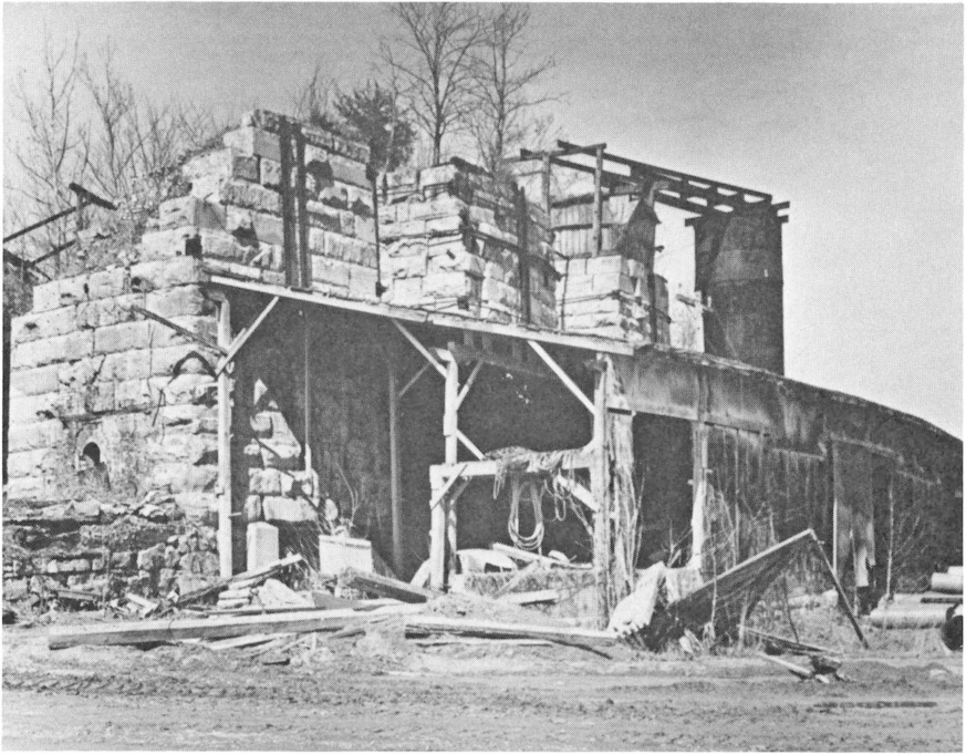
Figure 15. Abandoned vertical lime kilns used before 1932 at the Hoosier Lime & Stone Co. quarry near Salem.
