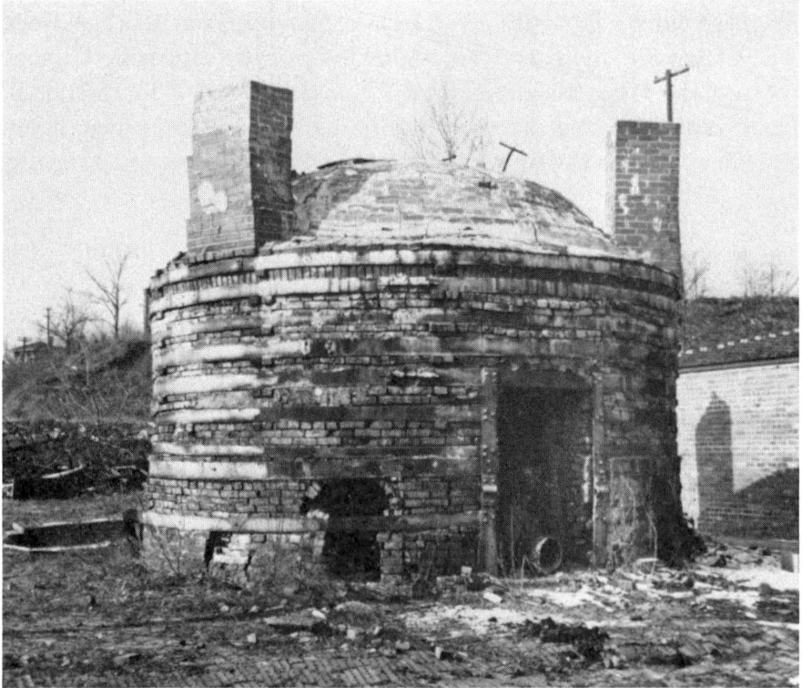
Figure 16. Beehive kiln used for burning lime at the Indiana State Farm near Putnamville, Putnam County, from 1924 to 1969.
